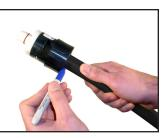
Stab pipe completely into fitting entrance.
